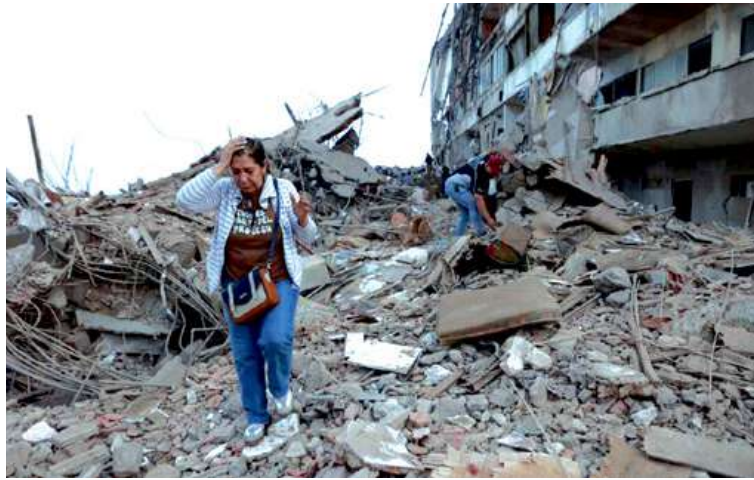
Residents walk amid the rubble of a building damaged in earthquakes the previous day in Catia La Mar, Venezuela. (Pedro Matthey/AP)
